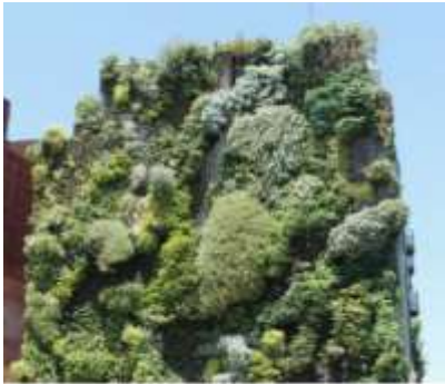
Continuous living wall system, Caixa Forum, Madrid, June 2013.
