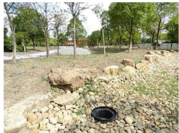
Rain garden under construction in the first round Sponge City Jiaxing (September 2016)
